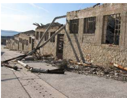
An abandoned building and a bent railing.
