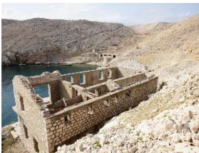
A roofless building above a cove.
