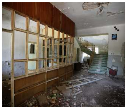
An abandoned corridor.
