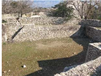
Dry-stone wall at the bottom of the pit.
